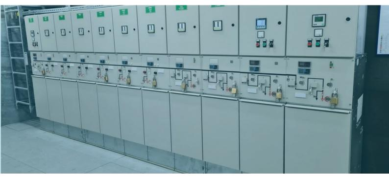
For the monitoring of transformer feeder panels it is of great advantage for the plant operators and plant constructors to realize the monitoring with fail-safe displays. This serves to quickly identify sources of failures in a de-energized state and therefore to a quick elimination of said failures.
